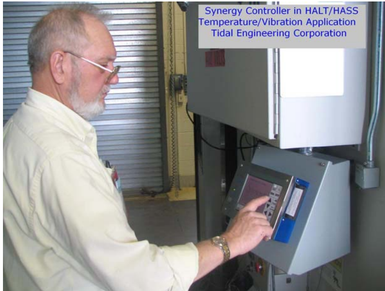
Figure 1, Synergy Controller Installation
